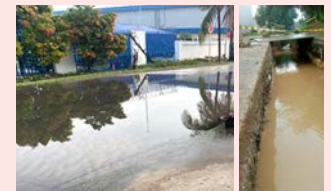
A flooded road
