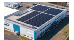
Solar power generation equipment of A.L.M.T. Corp. (Yamagata)
