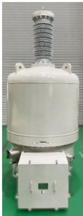
Photo 1. PVT for demonstration tests (66 kVA, 100 kVA)
