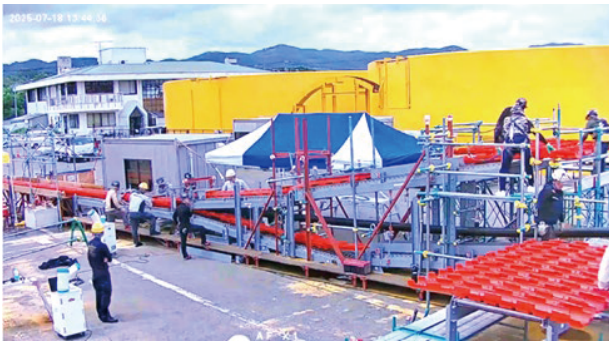
Photo 2. High-speed protection pipe laying, actual model
