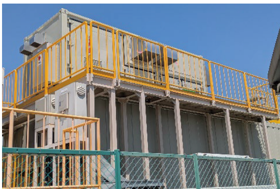
Photo 2. VRFB Prototype system
