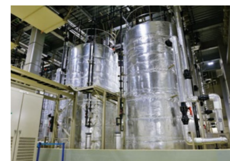
Electrolyte tanks in the building
