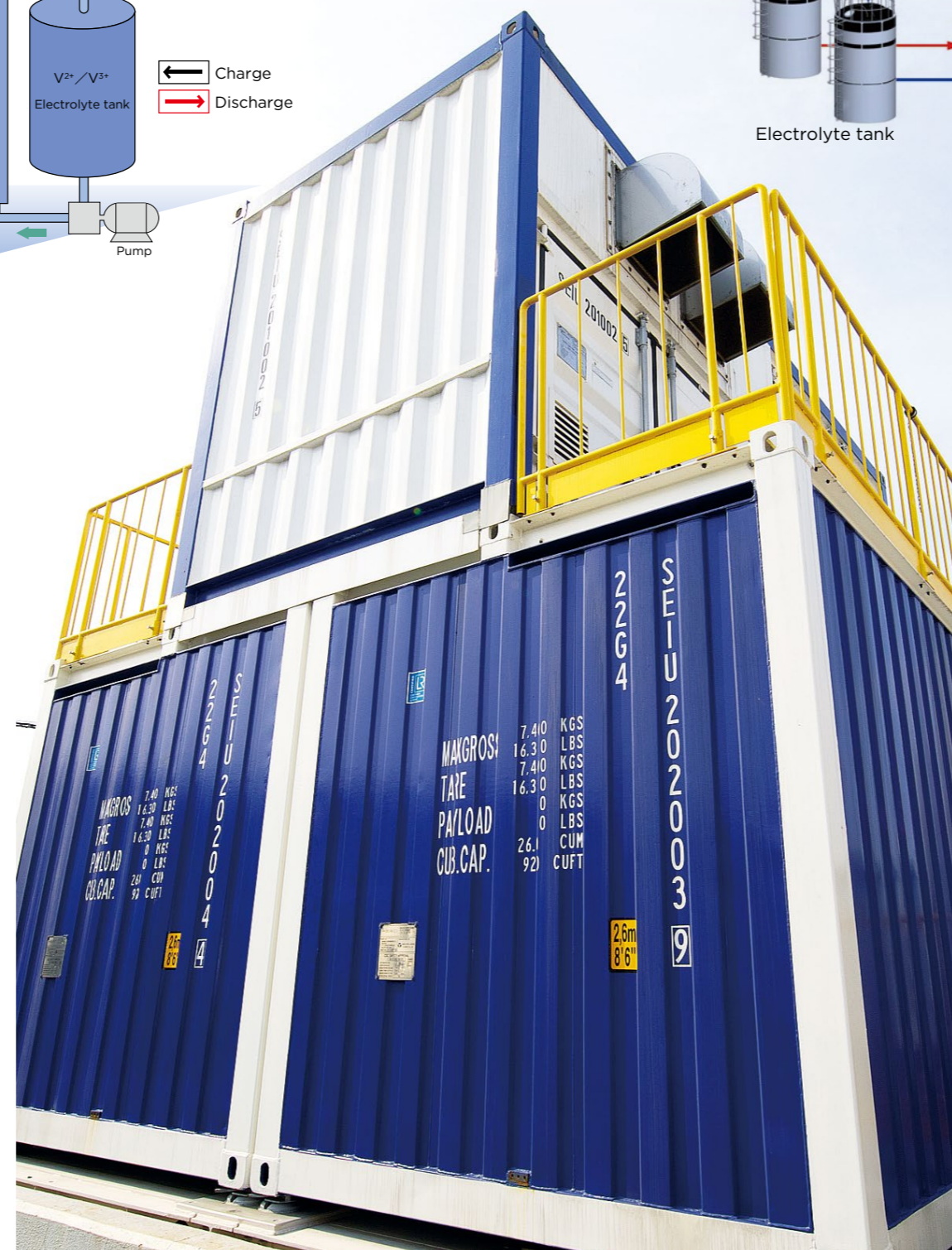
A redox flow battery consists of three devices: positive and negative electrolyte tanks installed on the first floor and cell stacks with electrolytic baths installed on the second floor.
