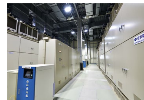
Battery cubicle
