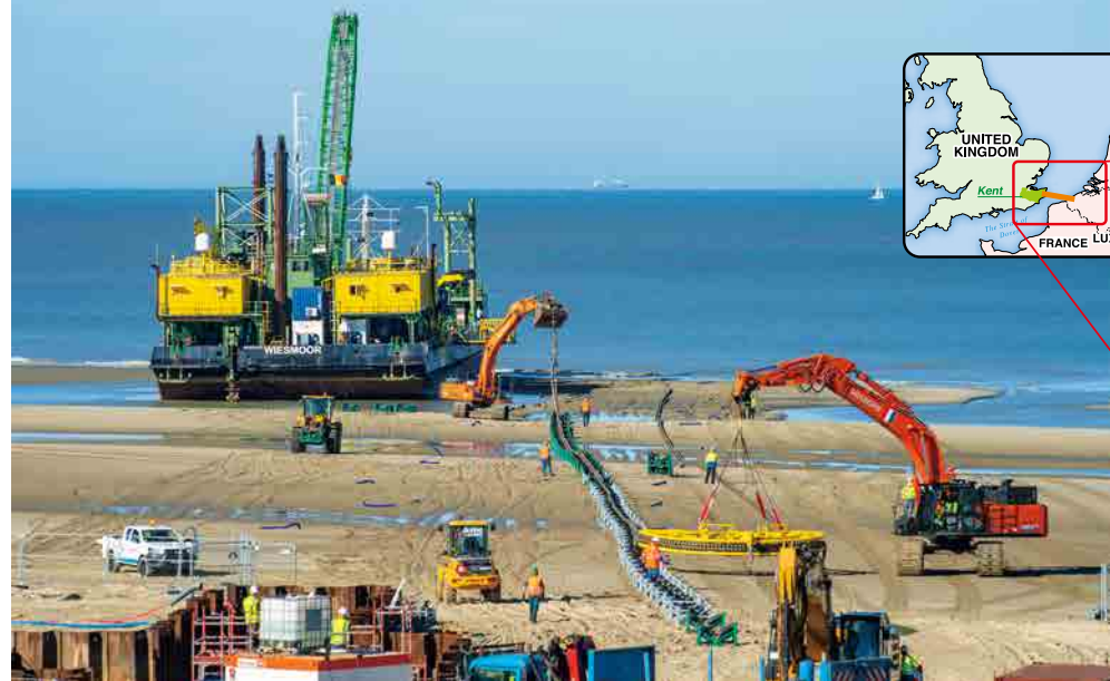
Cable laying on the Belgium beach side
