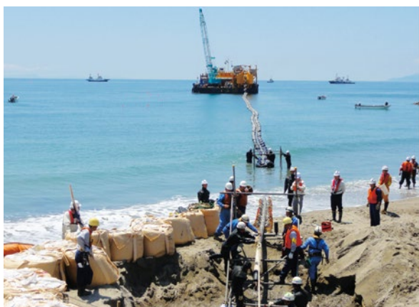
Cable installation for the Hokkaido-Honshu HDVC Link
