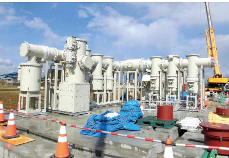
Construction of a grid connection switching station
