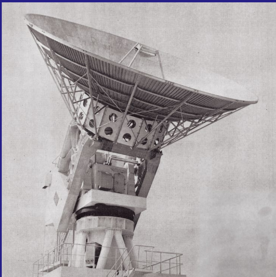
Parabolic antenna for a Syncom satellite, installed in Kashima, Ibaraki Prefecture, to broadcast the Tokyo Olympic Games to the U.S.
