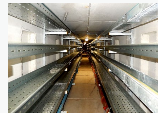
MCF-equipped underground tunnel in city of L'Aquila
