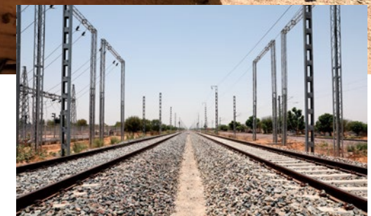
Orderly rows of poles are erected alongside rails before installing contact wires on the railroad
