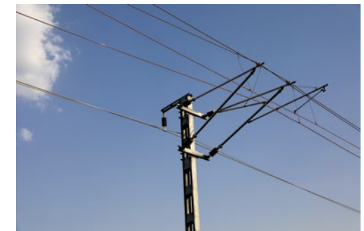
Wires and a pole supporting them to electrify the railroad
