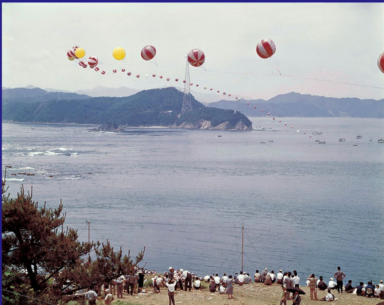
Laying a power transmission line to the opposite bank using balloons
