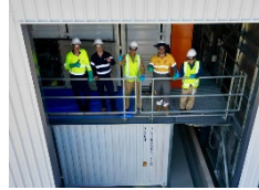
Energy Queensland 750kWh Electrolyte Production
