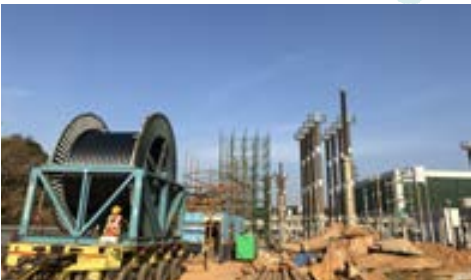
Cable installation site in India
