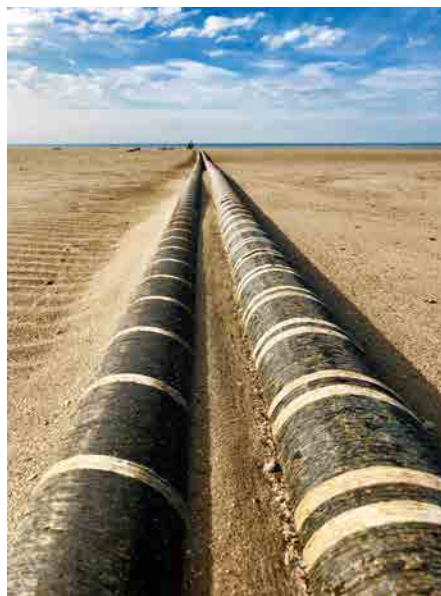
Nemo Link interconnector cables to be installed between UK and Belgium (before cable burial)
