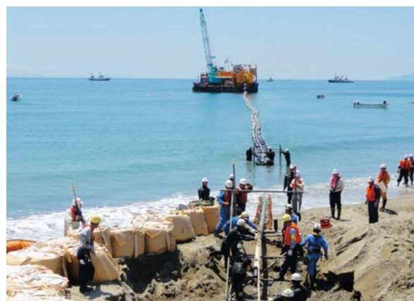
Cable installation for the Hokkaido-Honshu HDVC Link
