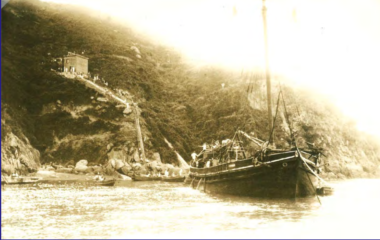
An end of the cable pulled up to Shisakajima
