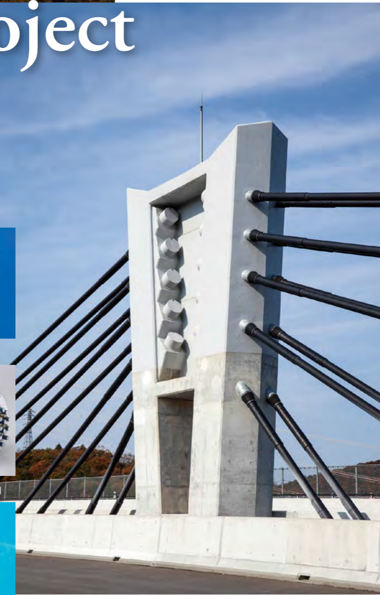
Anchorage zone of stay cables at pylon
