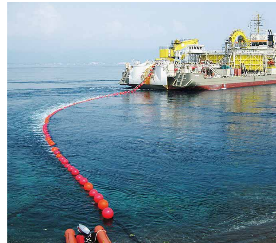
Submarine cable installation under high tidal current by DP-II vessel "Ndurance" in Bali Strait (by courtesy of VBMS)
