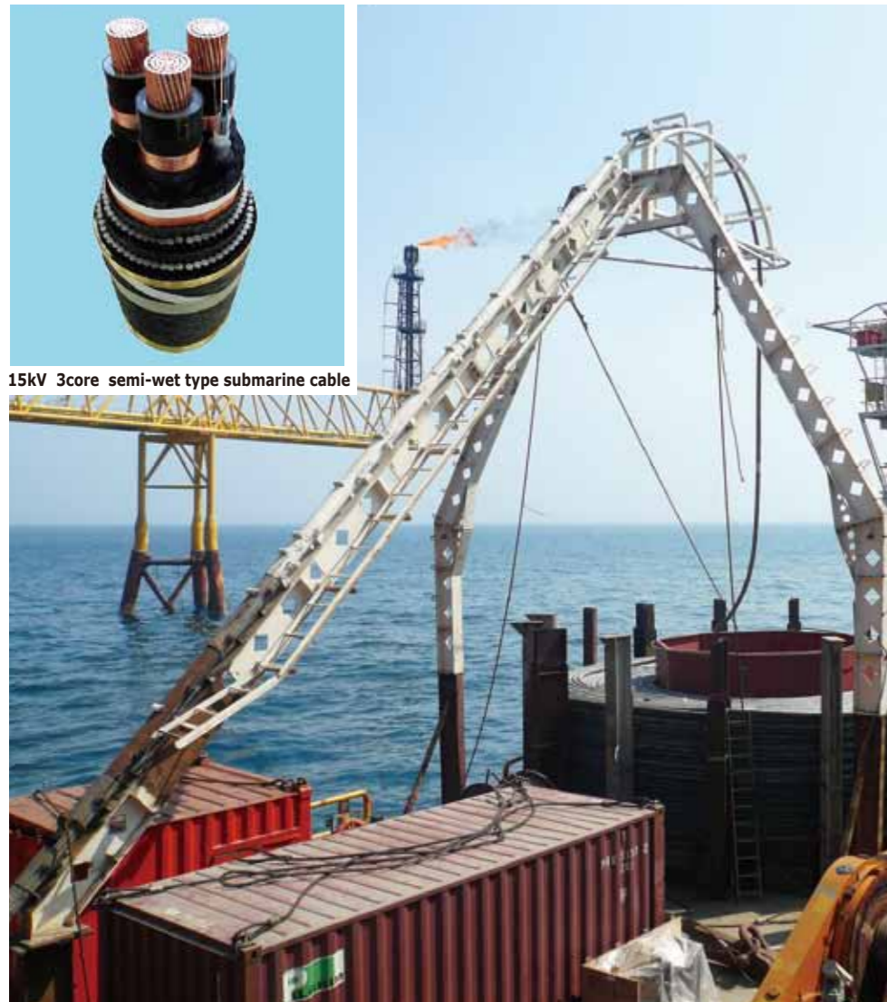
Unloading of MV submarine cable for oil platform
