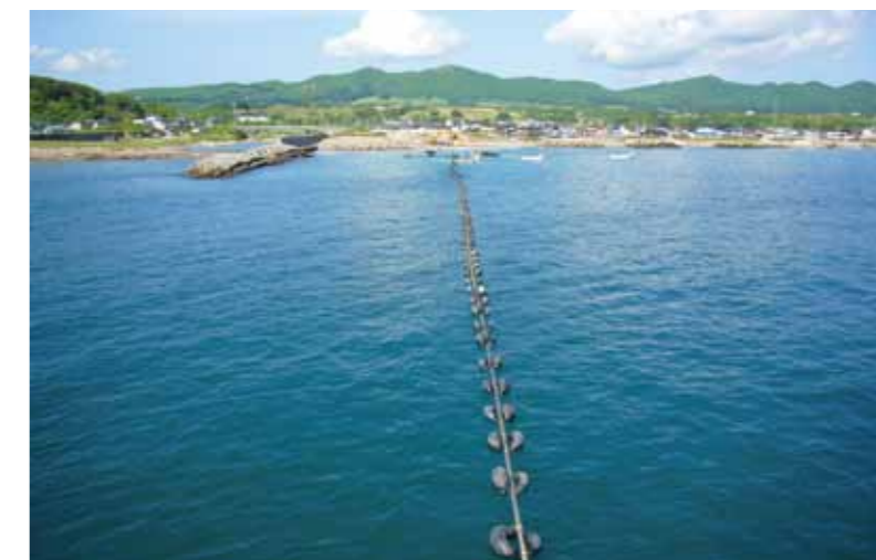
Cable installation of DC250kV XLPE cable in Hokkaido
