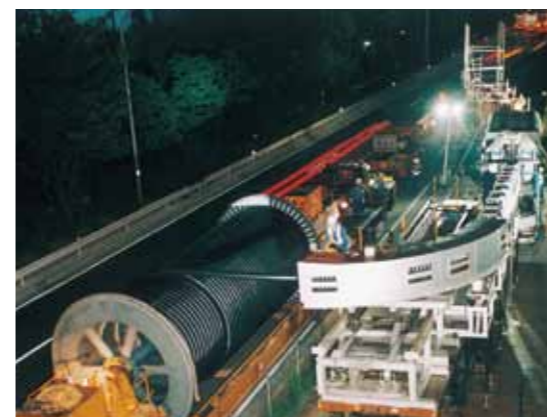
500kV XLPE cable installation work in Shinkeiyo Toyosu Line in 1996
