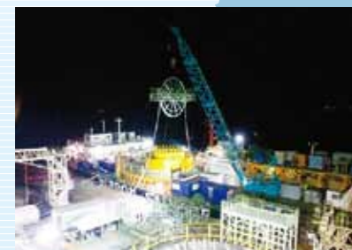
Loading on cable laying Barge for Russky Project
