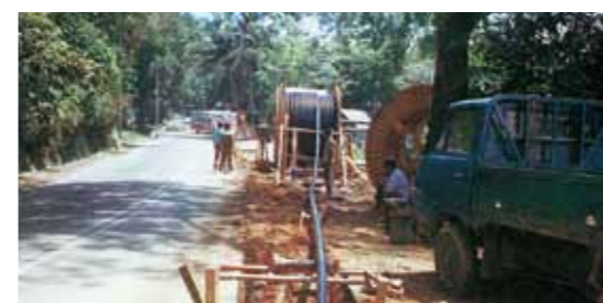
Direct burial cable installation work in Singapore
