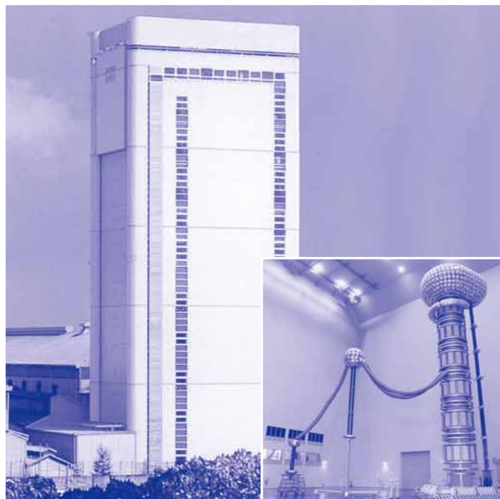
VCV tower in Osaka Works
