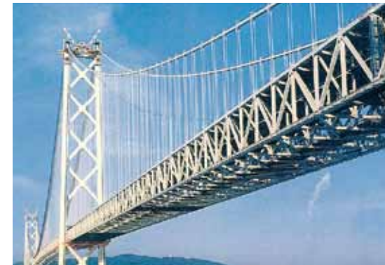
77kV XLPE cable installed on the world's longest bridge in 1998
