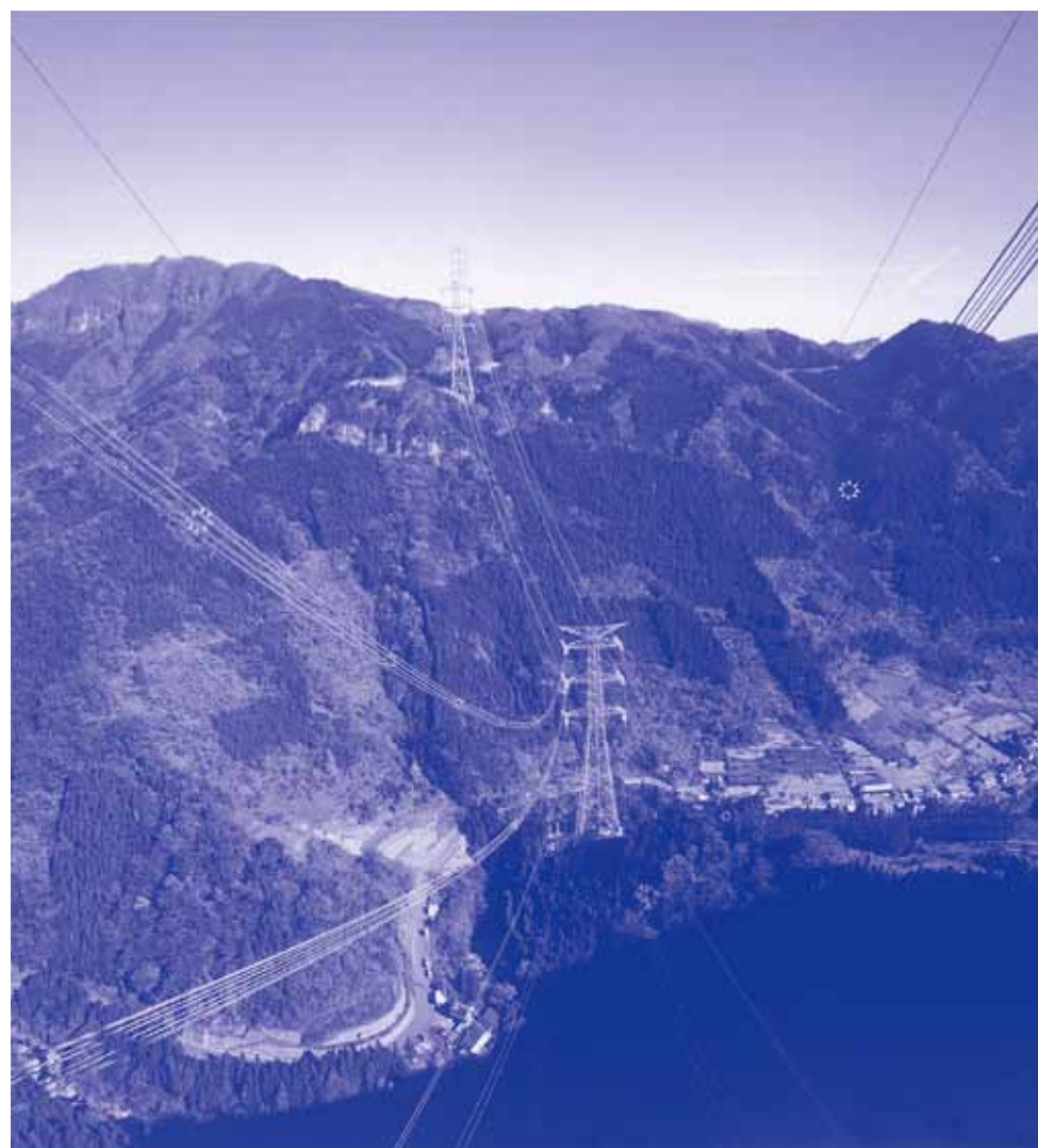
500kV transmission line using Aeolian noise suppressed conductor (NS-TACSR)
