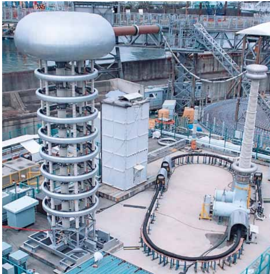
Electrical test laboratory at SEI's factory
