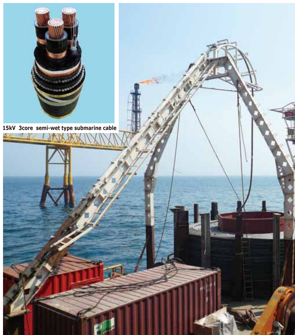
Unloading of MV submarine cable for oil platform
