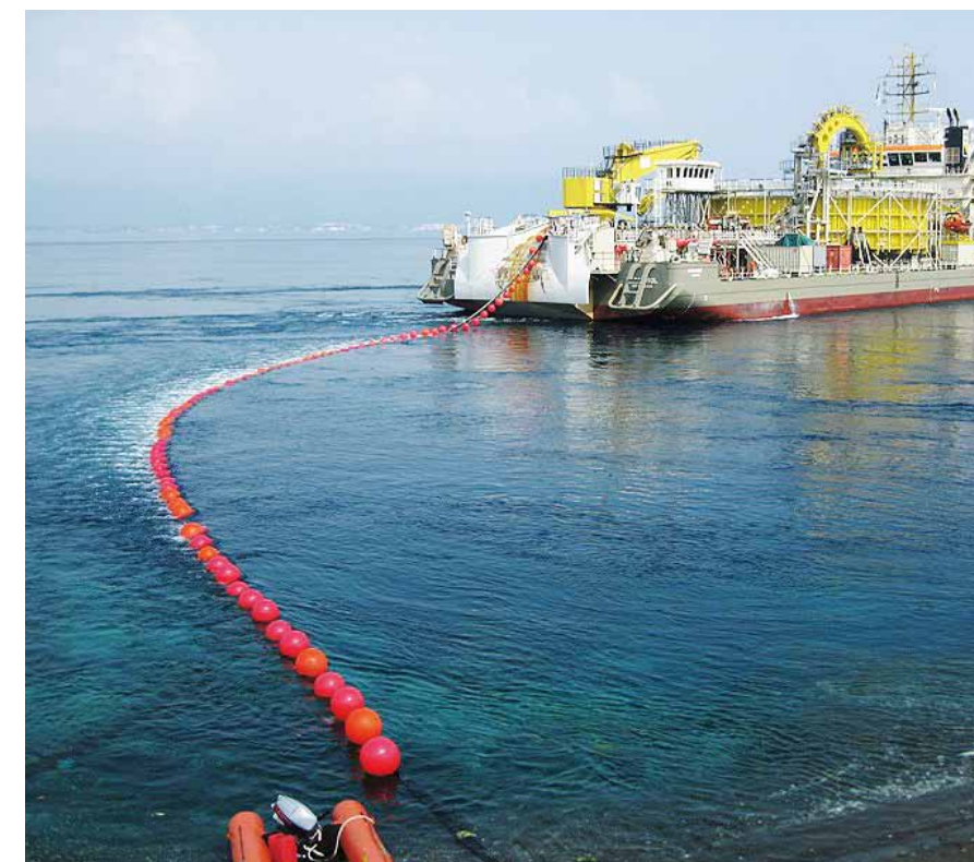
Submarine cable installation under high tidal current by DP-II vessel "Ndurance" in Bali Strait (by courtesy of VBMS)
