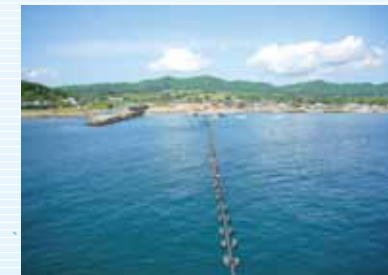
Cable installation of DC250kV XLPE cable for Hokkaido-Honshu Project
