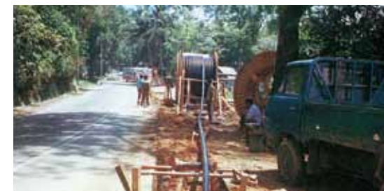
Direct burial cable installation work in Singapore
