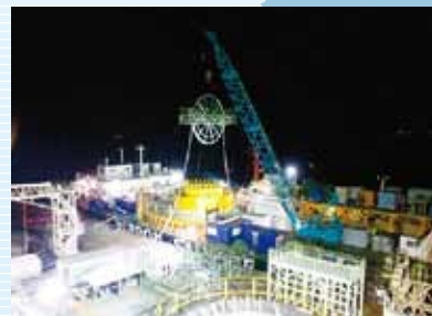
Loading on cable laying Barge for Russky Project
