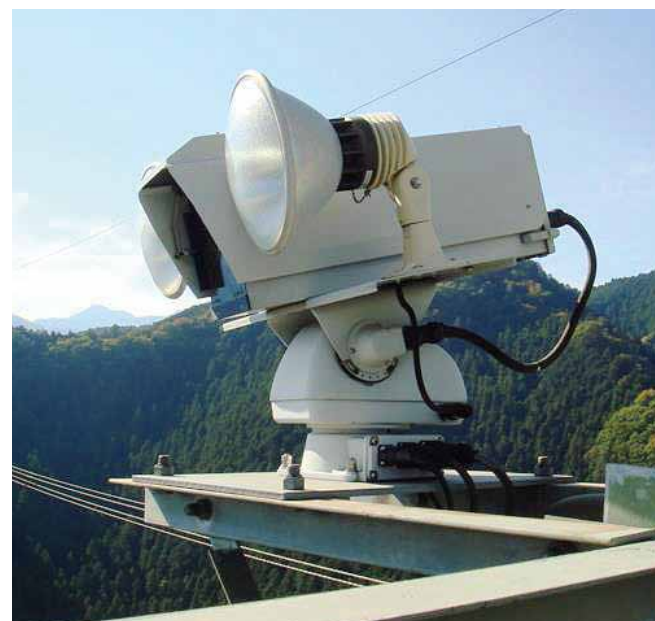
Controllable camera for monitoring overhead lines
