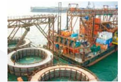
Off-loading power cable for transshipment for Lamma Project
