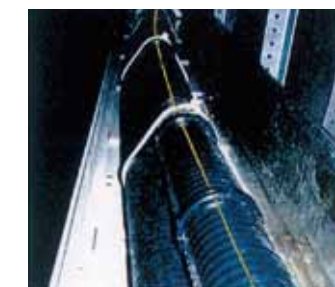
Cable temperature monitoring by Fiber-Optic Sensor
