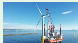
Photo courtesy of Akita Offshore Wind Corporation
