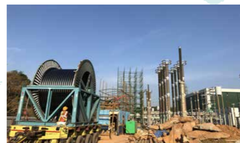
Cable installation site in India
