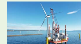
Photo courtesy of Akita Offshore Wind Corporation
