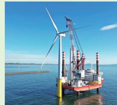
Photo courtesy of Akita Offshore Wind Corporation
