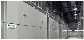
Floor 2: Cell stack and heat exchanger
