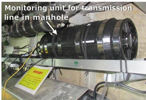
Photo 3. Monitoring unit for transmission line in manhole
