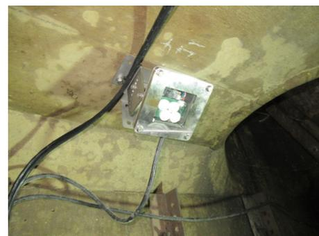
Photo 2. Example of camera installation in manhole
