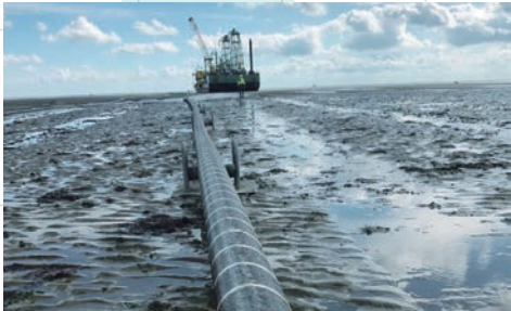
Submarine cable being installed
