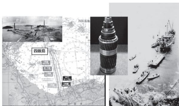
Photo 1. 11 kV submarine cable installed between Niihama and Shisakajima
