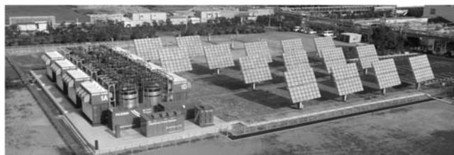
**Photo 1.** Outlook of a megawatt-class electric power generation/storage system
