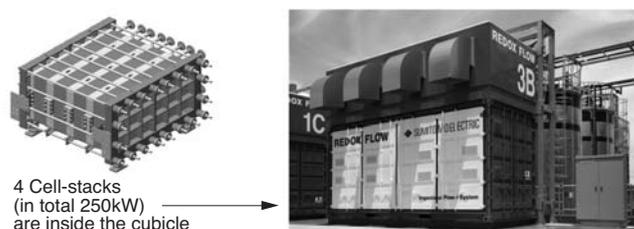
**Photo 2.** The new cell stacks and the battery cubicle
