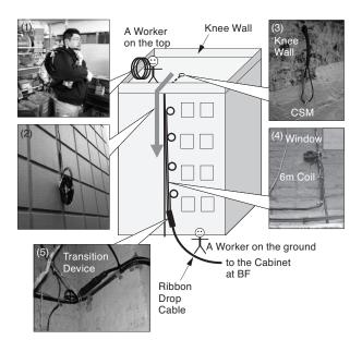
Fig. 8. Cabling network of field trial for small MDU
