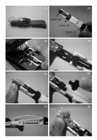
Photo 4. Outline of assembly procedure of LC connector for Ø0.9 mm fiber
