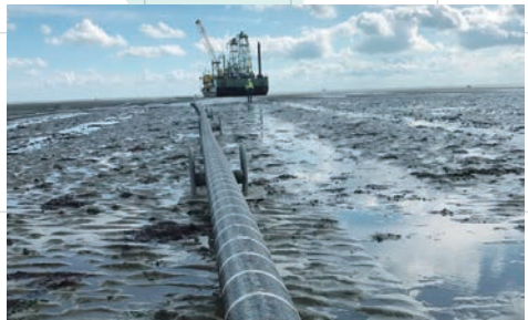
Submarine cable being installed
