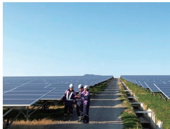
Construction work of a mega-solar system
