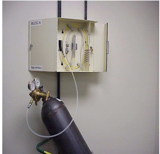
Figure 8 Ready Nitrogen Bottle at Entry Point FTU
