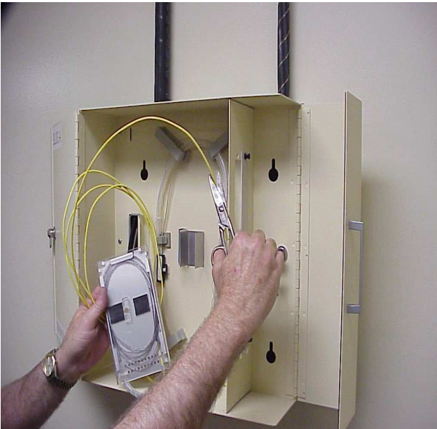
Figure 7 Remove Fiber Termination Hardware at both FTUs
