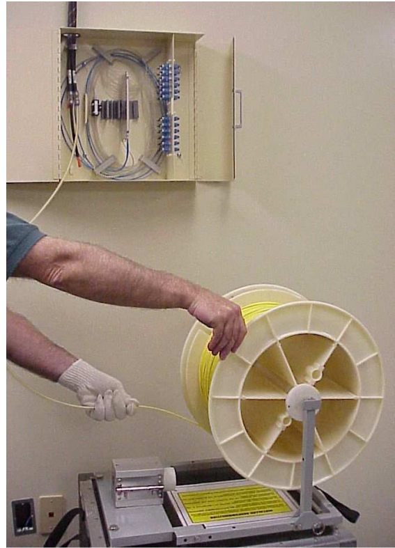
Figure 2 Blow Fiber Bundle Out of Damaged Tube and onto Empty Reel
